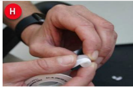
Wrap the Elbow fittings with new Teflon tape
