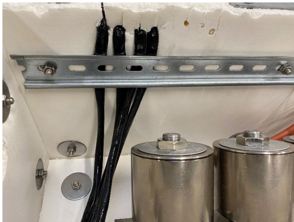
Figure 4-2, Multiplexer Cable Management
